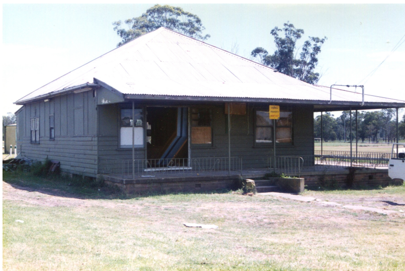
Above : The Greenhouse. Ironically, this photo was taken literally one day before bulldozers arrived to flatten the site in 1999.
