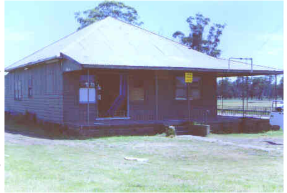
The Greenhouse—Photographed one day before it was finally demolished to make way for the new Olympic Precinct.
